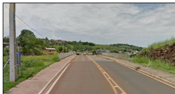
Figura 5.30 – Travessia Jamile Dequech
