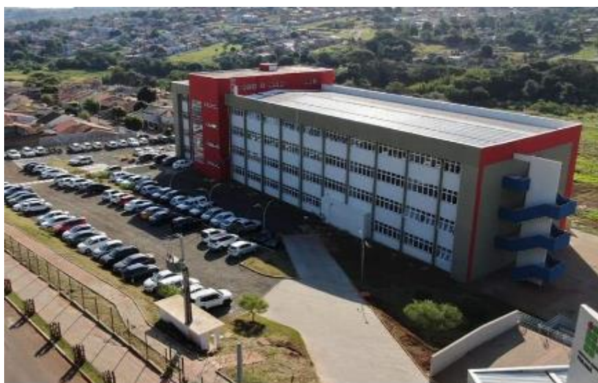
Image 6 - IFPR's physical infrastructure in Londrina
