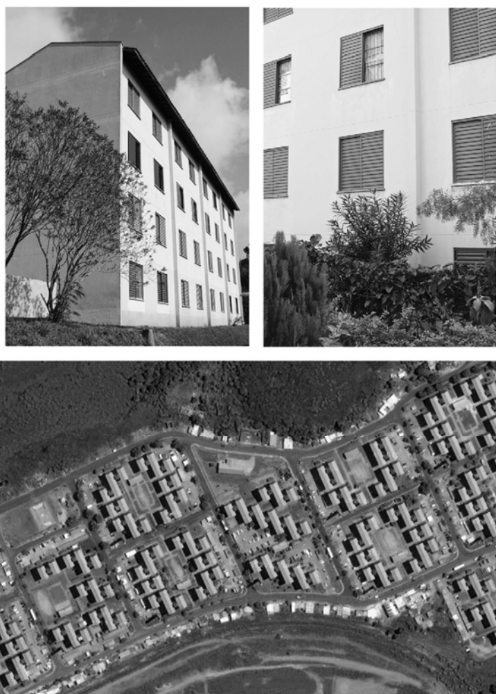
Fig. 3. Views of multi-family social housing projects based on four storey walk-up apartment blocks in the region of the city of Campinas, SP, Brazil.
