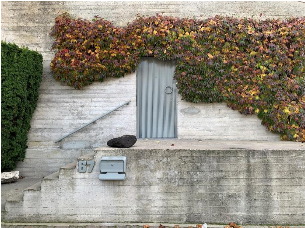
Figura 52: House Merckaert, Geraardsbergen, Belgium, 1978
