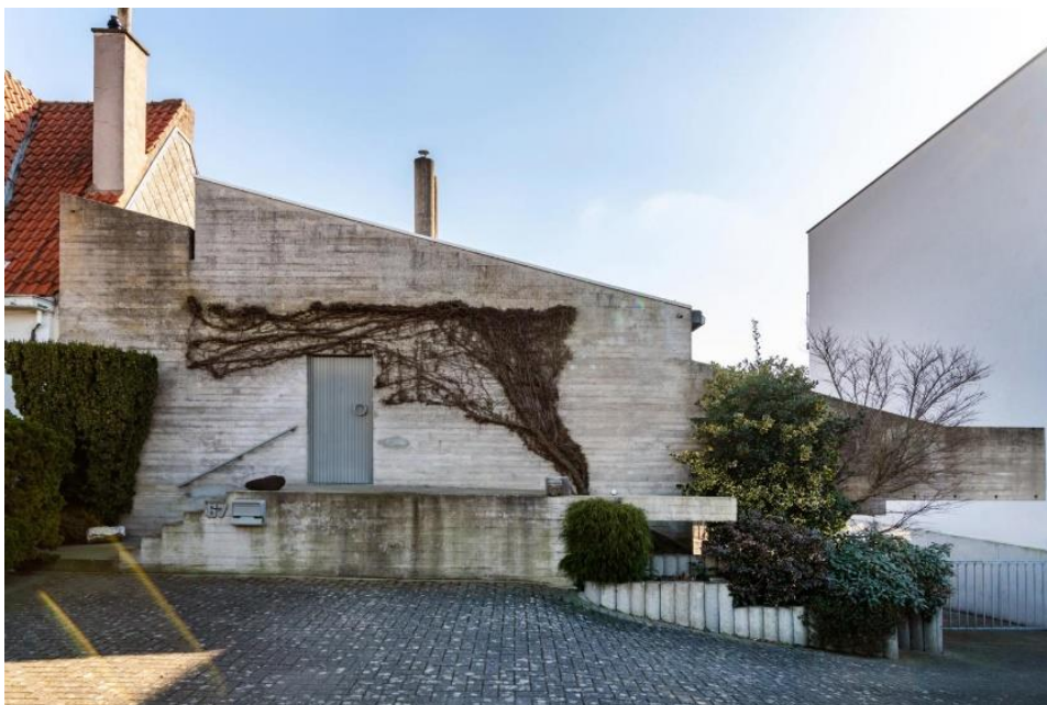
Figura 49: House Merckaert, Geraardsbergen, Belgium, 1978
