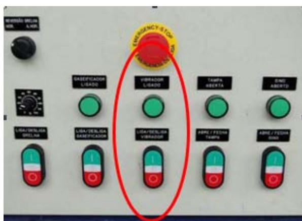
Figura 26 – Botoeira “Liga/Desliga Vibrador”
