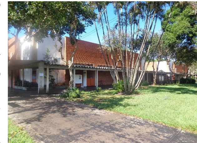
Figura 95 - CCH, Bloco A (mai.2017)
