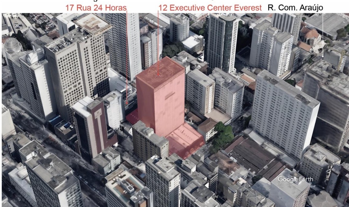
Figura 14- Vista aérea: Executive Center Everest
