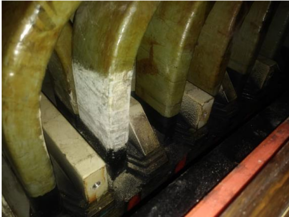
Figure 76 – Corona repair process in UG3 in 2019.
