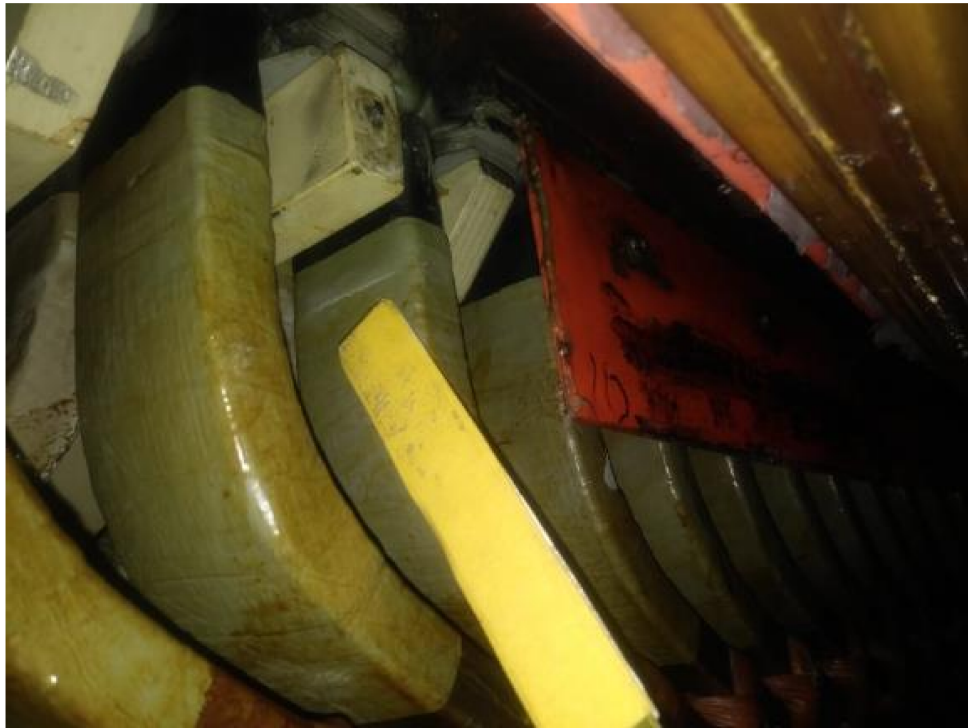
Figure 75 – Corona spots identified in UG3 in 2019.
